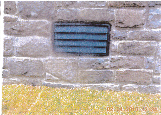
CRAWL SPACE DOOR SYSTEMS FLOOD VENT MODEL 816CS TYPICAL OF 5
